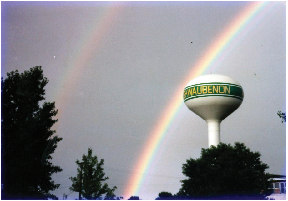
The water tower is a familiar skyline site at Lois Aubinger Park.
