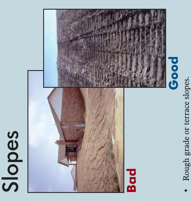
Break up long slopes with sediment barriers, or under drain, or divert stormwater away from slopes.
