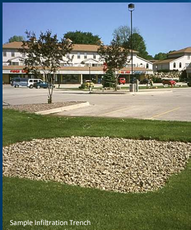
Sample Infiltration Trench
