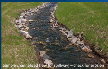
Sample channelized flow (or spillway) - check for erosion
