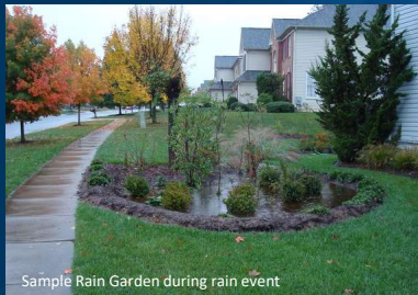
Sample Rain Garden during rain event
