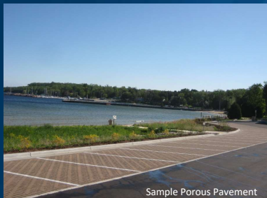
Sample Porous Pavement
